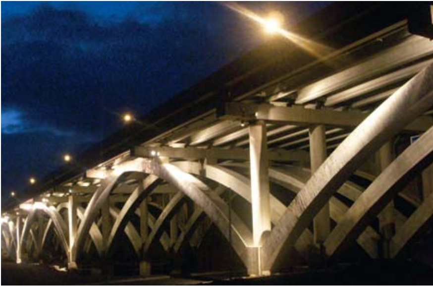
The new 1345-ft precast concrete arched bridge over the Fox River along I-88 in Illinois, designed to add lanes alongside an existing arched bridge, proved so successful that the project was extended to replace the original bridge, too.
